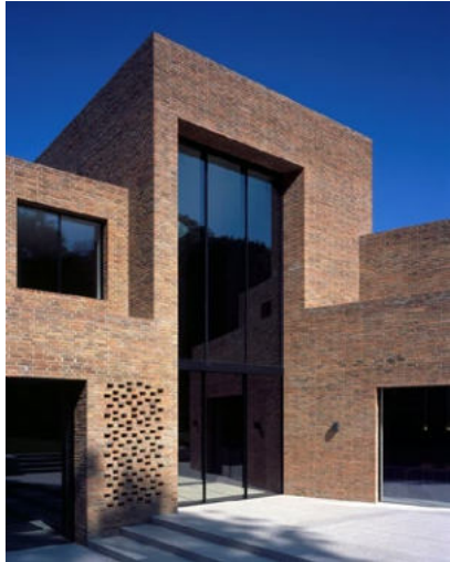
Precedent Example of brickwork
