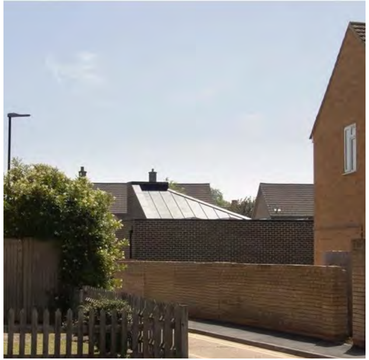
Fig.5.7 - Backland massing approach. The proposal for a two bedroom home is located in the former garden of a house in Pollards Hill, Mitcham. The proposal is single storey and designed to avoid overlooking to and from neighbouring homes whilst being discreet in it's massing. (Nineteenth Road, Pollards Hill by Decent Goodfellow Architects )
