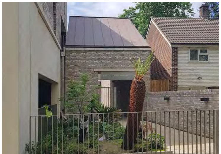
Fig.5.13 - Entrance to GP surgery is marked out by a form in keeping with neighbouring properties. [Credit: Panter Hudspith]
