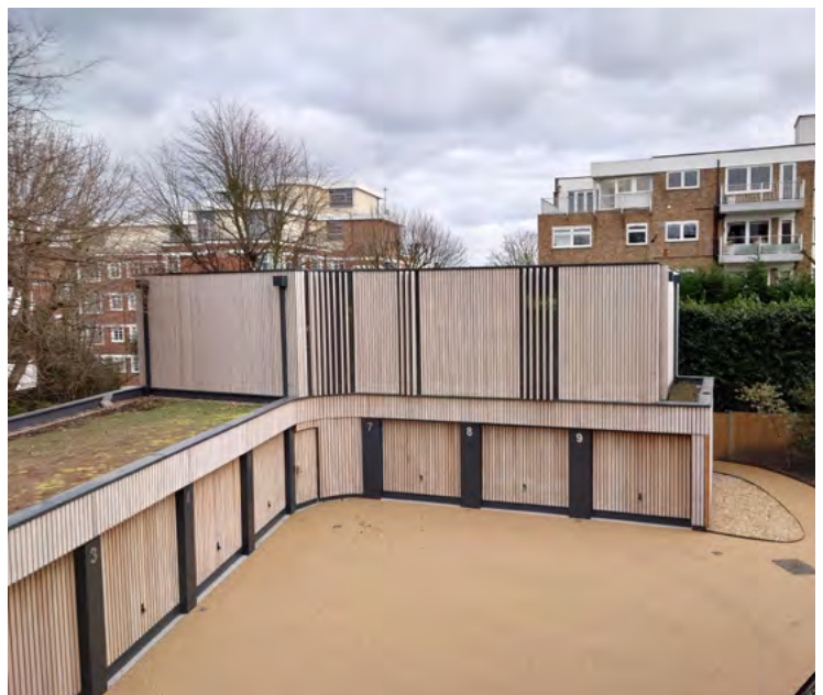
Fig.5.27 - Extensive green roof and improved pedestrian and vehicle space. [Credit: Future Merton]
