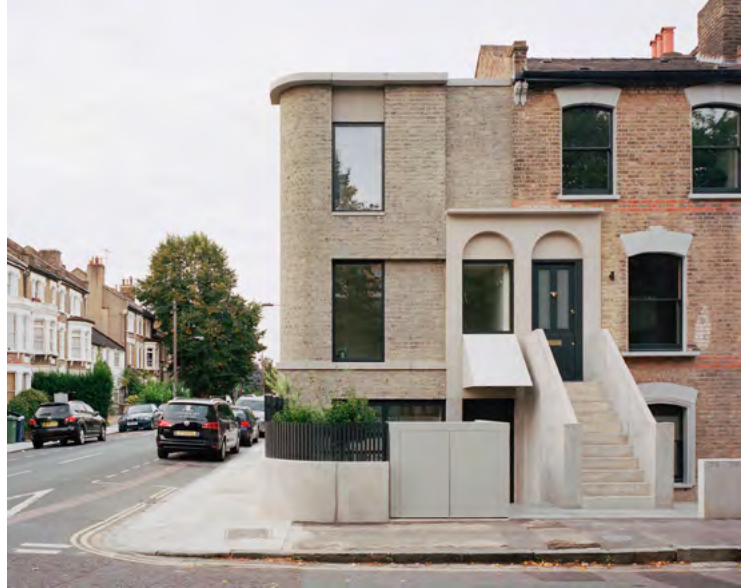
Fig.7.34 - This extension to an existing terrace promotes a sense of safety by incorporating defensible space fronting the street. (Corner House, Southwark by 31/44 Architects ) [Credit: Rory Gardiner]
