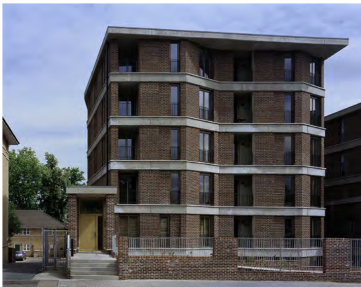
Fig.5.12 - The entrance of these villa blocks protrude towards the street and stand higher than the concrete banding marking each level. This creates a welcoming entrance that is distinct from other openings in the building fabric. (Finsbury Park Villas, Haringey by Sergison Bates Architects ) [Credit: Stefan Müller]
