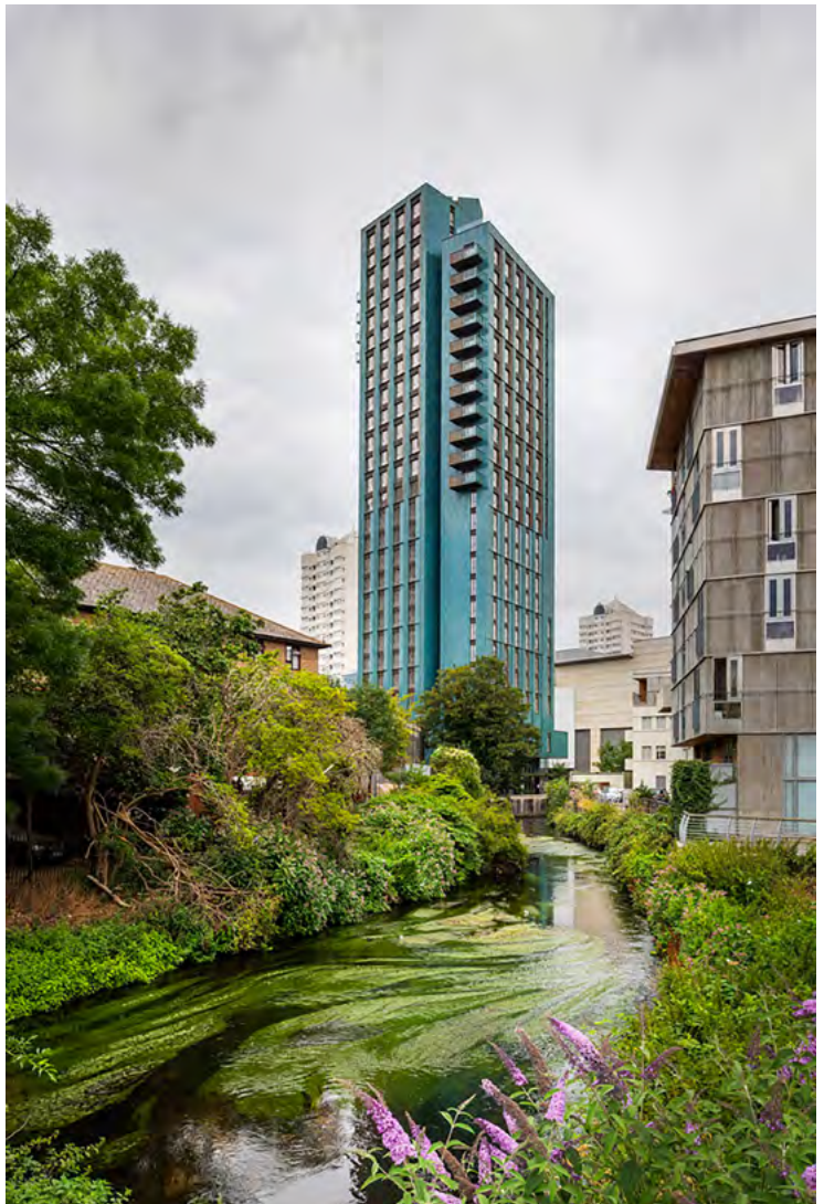
Fig.5.30 - View to tower from the river Wandle. [Credit: Simon Kennedy]
