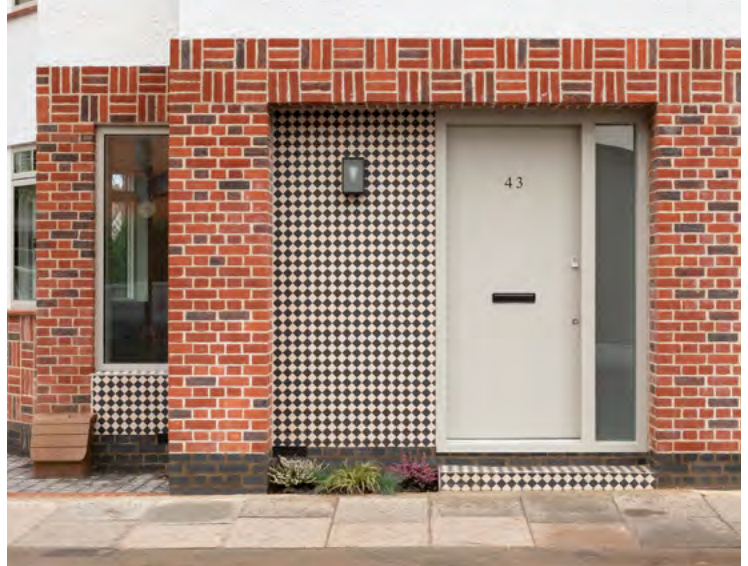
Fig.8.6 - New-build house references the terracotta brickwork as well as the Victorian tiling to front entrances of the neighbouring terrace homes. (Lucien road by Harp & Harp Architects ) [Credit: Harp & Harp Architects]
