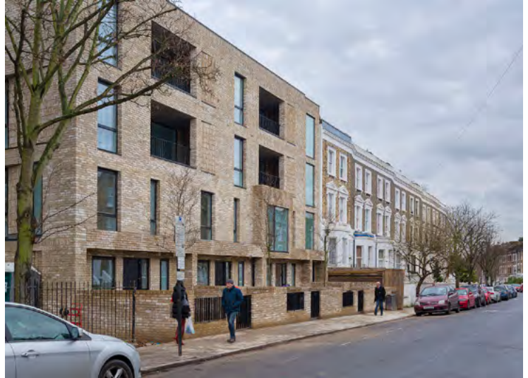
Fig.7.30 - A mix of home types in a compact building, it provides duplexes at street level with flats above. (Vaudeville Court, Islington by Levitt Bernstein ) [Credit: Tim Crocker]
