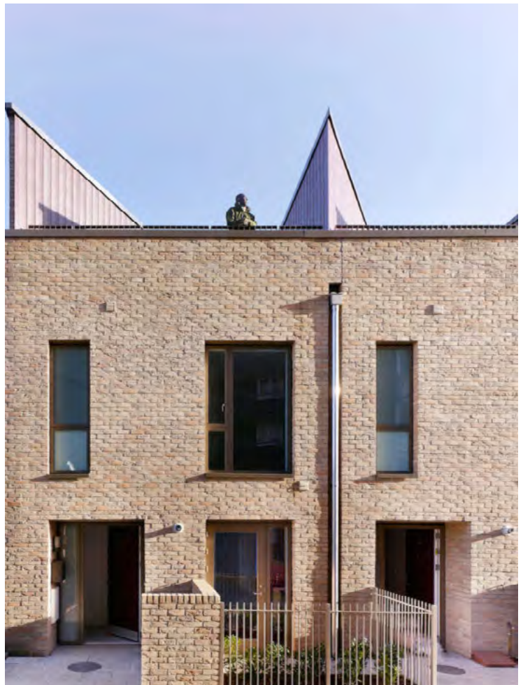
Fig.5.8 - View of front elevation and defensible space. [Credit: Bell Phillips Architecture]
