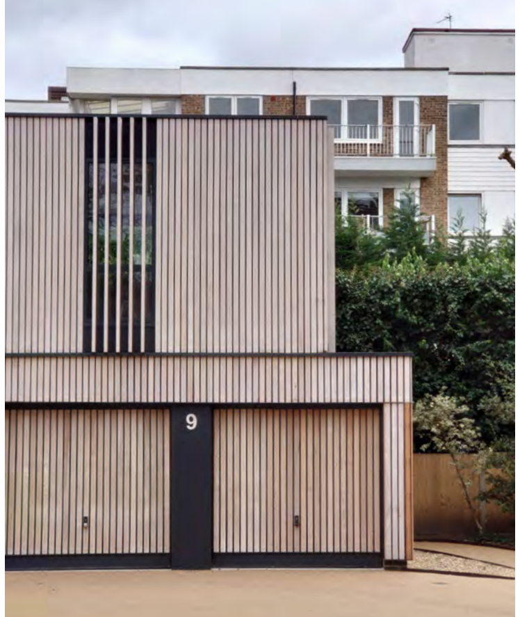
Fig.5.26 - Home above garages [Credit: Future Merton]
