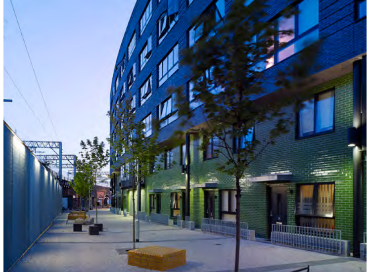
Fig.6.15 - The new homes provide a dual aspect with living rooms and kitchens facing the busy railway line opposite. This helps position bedrooms on the quieter side of the building. (Mint Street Housing, Tower Hamlets by Pitman Tozer Architects ) [Credit: Kilian O'Sullivan]
