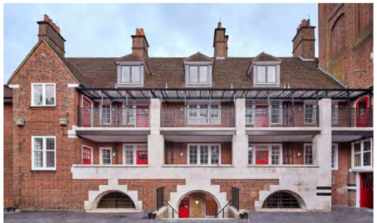
Fig.5.5 - Sensitive restoration of existing Grade II* fabric. [Credit: Kilian O'Sullivan]
