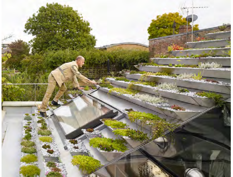
Fig.8.1 - This backland development meets the principle of 'no net loss in green cover' by incorporating planters on the roof to allow for a diversity of plants and therefore an increase in biodiversity. (Garden House by Hayhurst and Co Architects ) [Credit: Kilian O'Sullivan]
