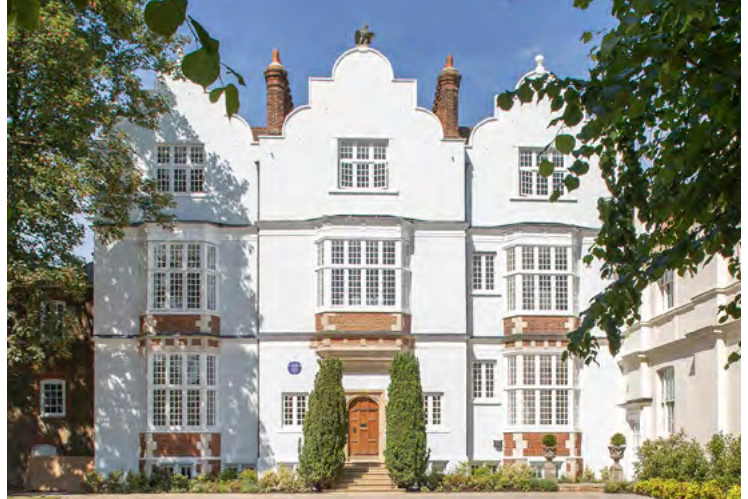
Fig.5.2 - A sensitive conversion and extension of a listed building to provide new homes. (Eagle House by Michaelis Boyd Associates ) [Credit: Octagon Developments]
