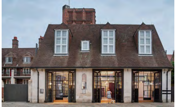
Fig.5.3 - Former engine bays converted into living space. [Credit: Kilian O'Sullivan]
