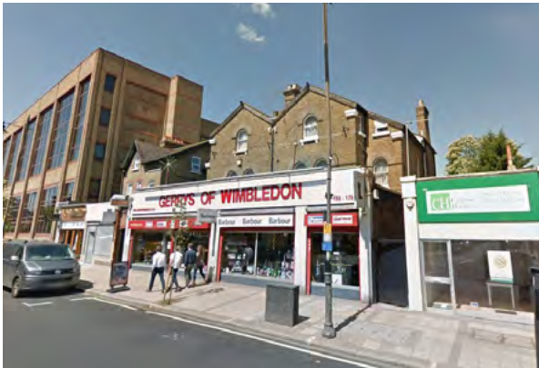
Fig.3.7 - Neptune House, Wimbledon (Left: Before. Right: After)
