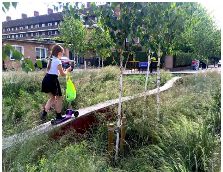
Fig.8.5 - Previously a road heavily used for children drop-off, Bridget Joyce Square, London, integrates sustainable drainage and play in the public realm. [Credit: London Wildlife Trust]
