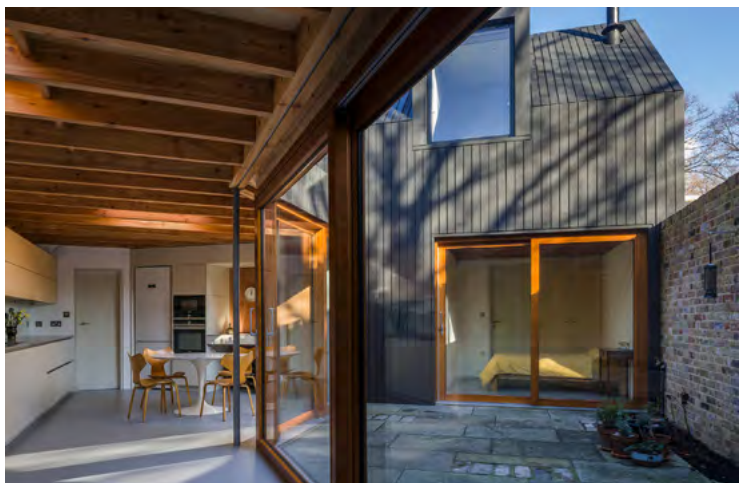
Fig.5.45 - A courtyard garden provide ample daylight to all rooms in the development
