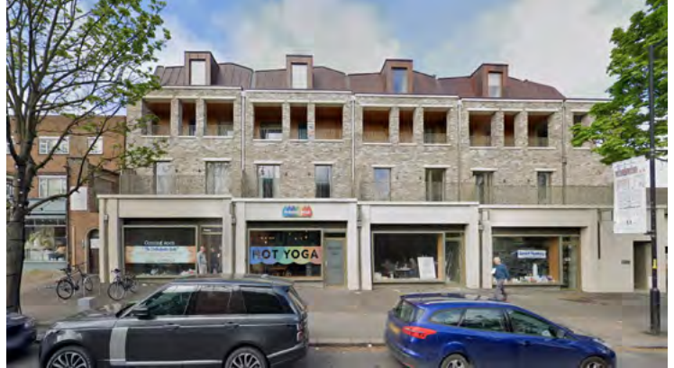
Fig.5.11 - Ground floor retail units continue the parade of shop fronts. [Credit: Panter Hudspith]
