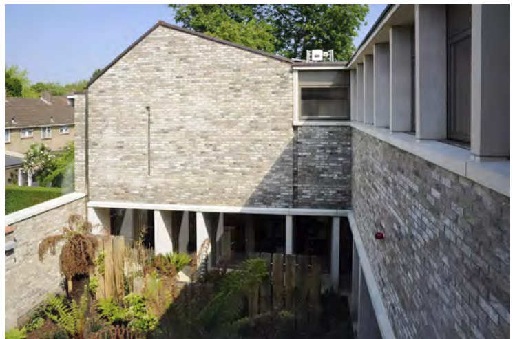
Fig.5.12 - Residents' access overlooking courtyard in the GP Surgery. [Credit: Panter Hudspith]
