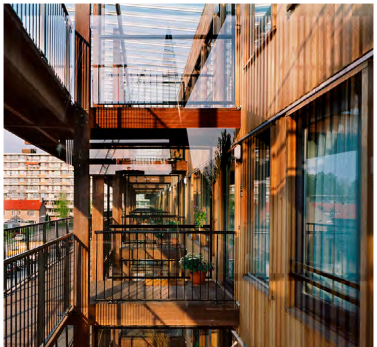
Fig.6.21 - Bridged gallery access provides semi public front garden and better privacy and daylight. (Koekoekspreuw, Amersfoort by KCAP ) [Credit: KCAP]
