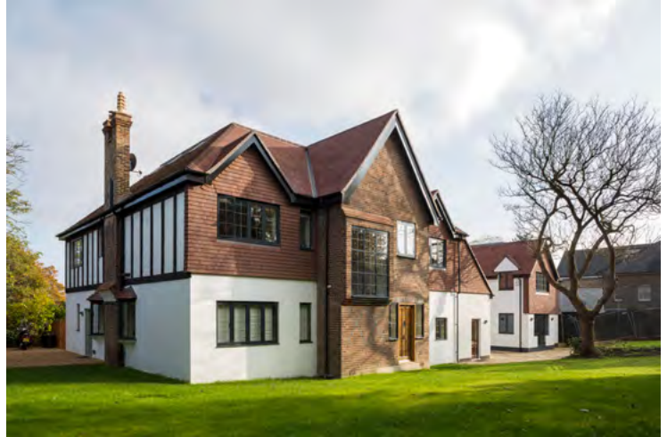
Fig.5.3 - Former engine bays converted into living space. [Credit: Kilian O'Sullivan]
