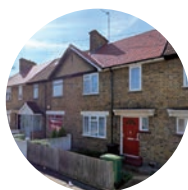
Municipal cottage housing
