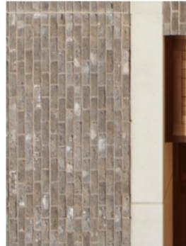
04 Pre-Cast Concrete Elements
