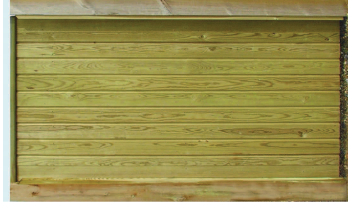
CLOSE BOARDED FENCE TO RAINBOW ESTATE
