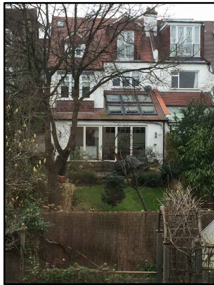
View from the second floor
