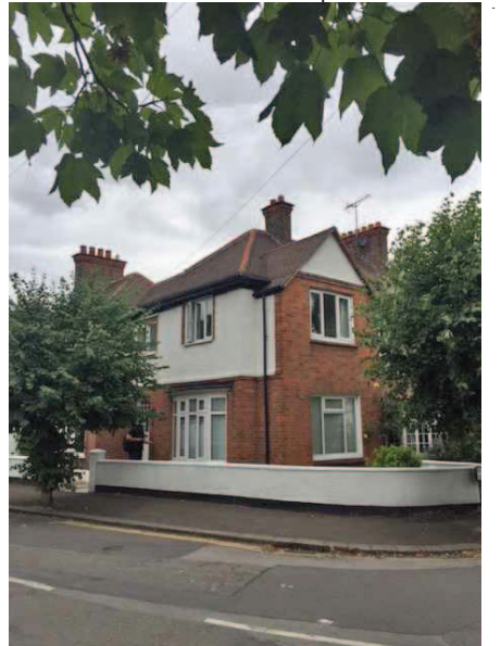
elevation to melbourne road
