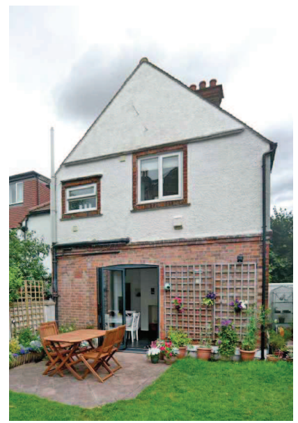
photo showing rear gable end to property
